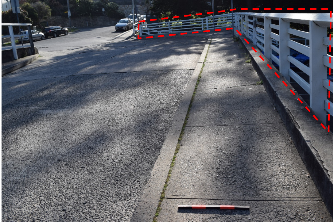
Figure 34: View of concrete road surface and footpath, and post and rail fence with diagonal top rail bordering bus zone on either side. Note: fencing to northern side of zone features additional members and is elevated (circled in red). (Source: City Plan Heritage).
