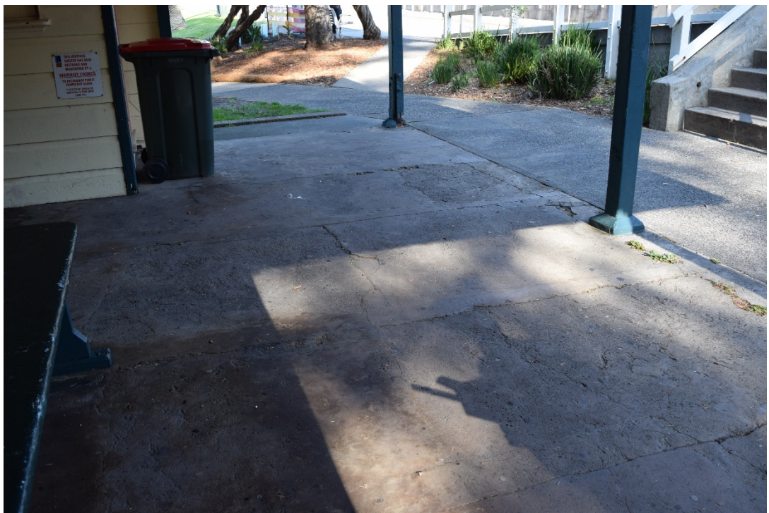
Figure 25: Modified ground levels between the tram shed and the footpath to allow for disabled access. (Source: City Plan Heritage).
