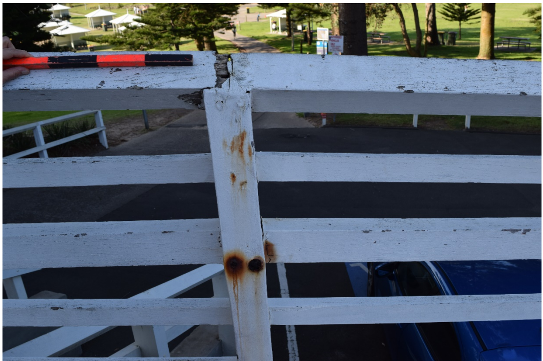
Figure 27: Post and rail fence indicating condition and evidence of previous repairs (Source: City Plan Heritage).
