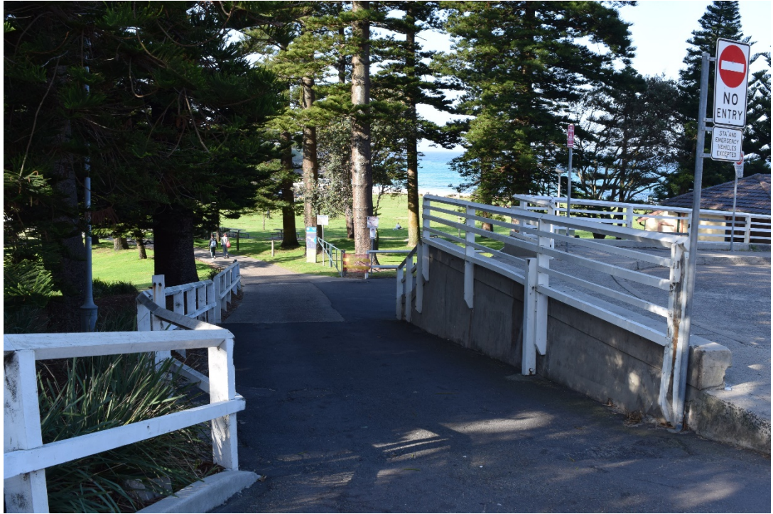
Figure 26: Entrance ramp to the disabled car park and Bronte Park with post and rail fence with diagonal top rail. Note: The fence to the right-hand side features additional horizontal members. It also forms the western boundary of the subject site (Source: City Plan Heritage).
