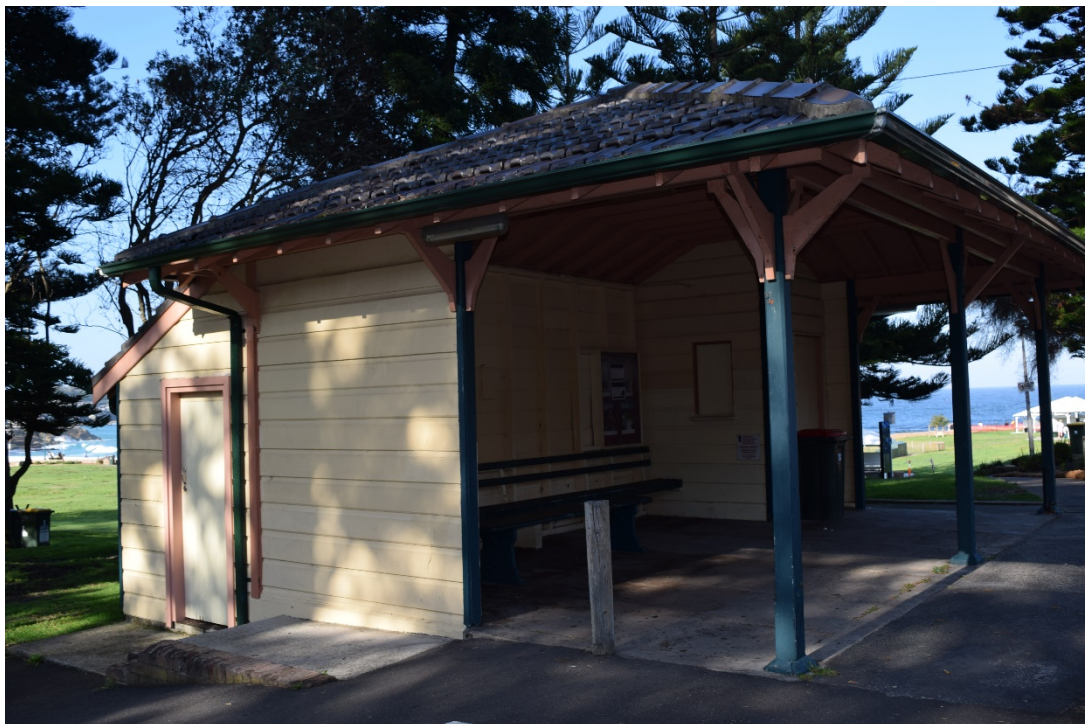
Figure 23: Timber-weatherboard former tram shed with lean to extension, terracotta roof tiles, timber bench, noticeboards and concrete floor. (Source: City Plan Heritage).
