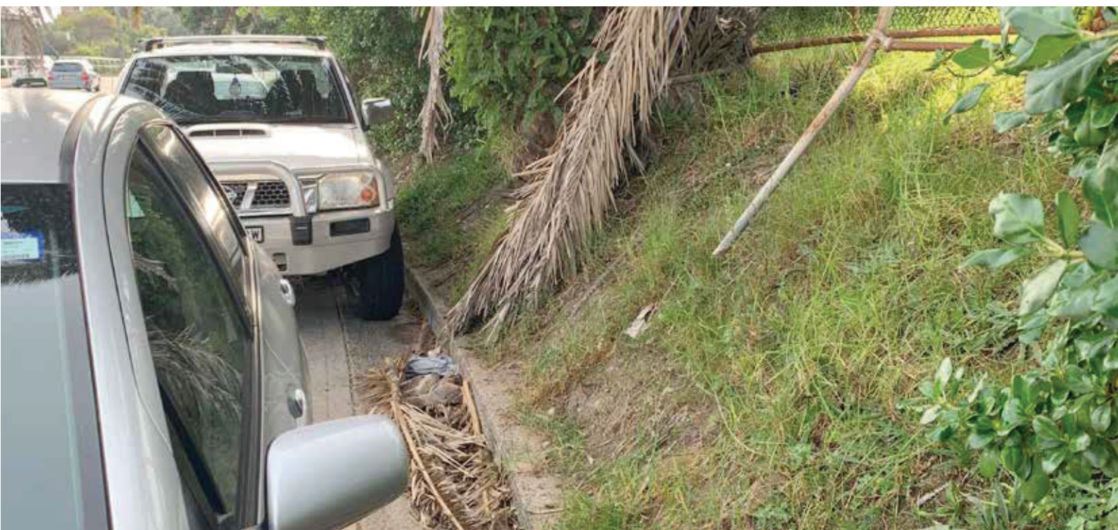
Image: Steep verge areas on Military Road will require localised earthworks and low walling to enable pedestrian path construction. To specific areas removal of parking is required to continue path
