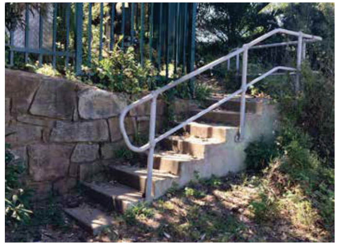
Image: Existing stairs are not compliant
