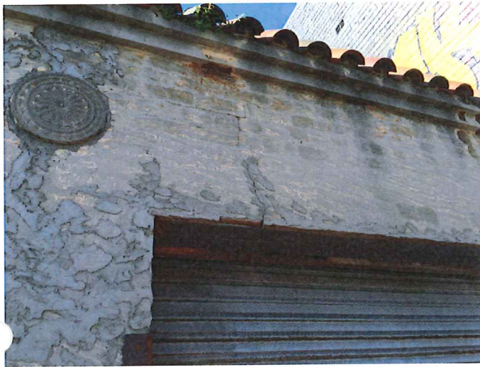
Photo 13 - Damage over garage door opening. Note repairs to previous damage as a result of corroded lintel.
