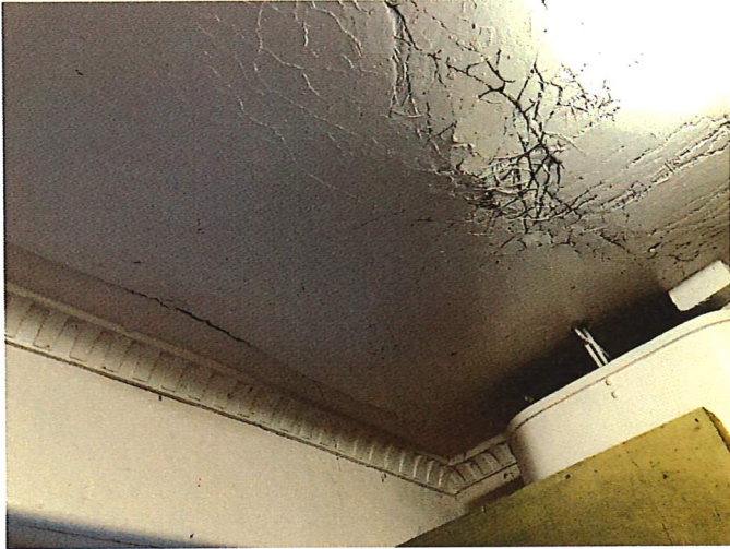
Photo 5 - Deteriorating ceiling to W/C of retail tenancy at 227 Bronte Rd
