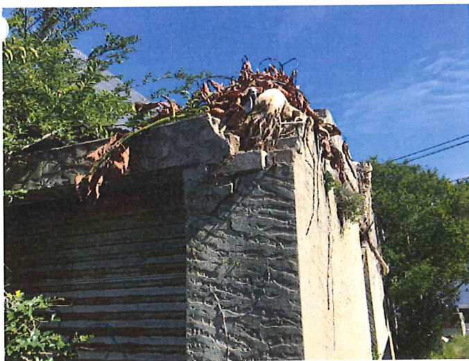
Photo 15 - Tree trunk growing within wall. Significant damage to wall and it would be anticipated that there significant damage to the floor and footings
