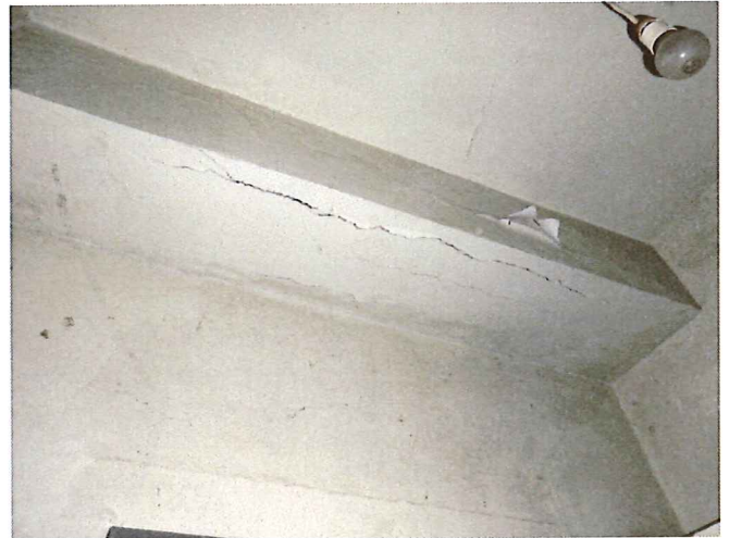
Photo 14 - Evidence of concrete cancer to the steel beams.
