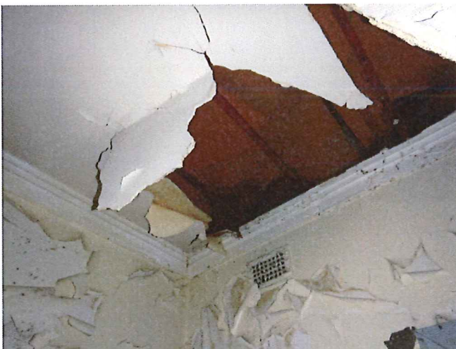
Photo 7 - Water damage to ceiling in unit 2
