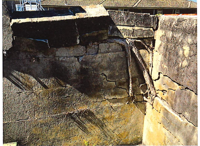
Photo 2 - Deteriorating balustrade
