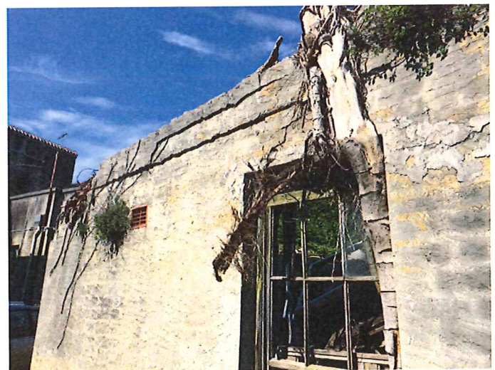
Photo 16 - Tree trunk growing within wall. Significant damage to wall and it would be anticipated that there significant damage to the floor and footings
