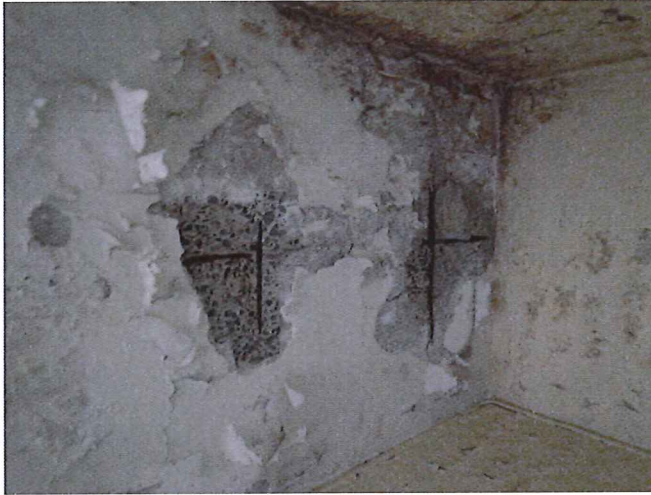
Photo 9 - Evidence of concrete cancer to suspended slabs. This is a significant issue throughout the building through all concrete slabs.
