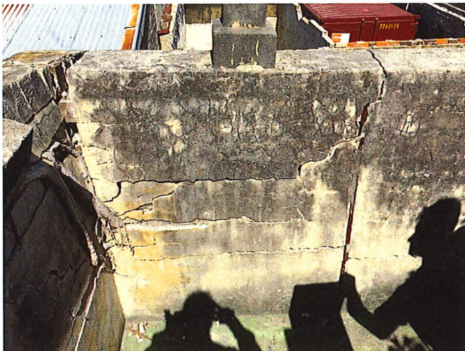
Photo 3 - Deteriorating balustrade
