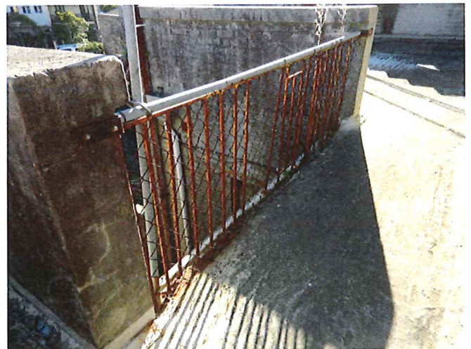
Photo 24 - Balustrade to upper level walkway is in extremely poor condition and needs to be replaced
