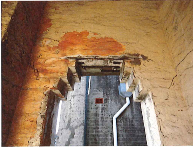
Photo 33 - Evidence of corrosion of lintels embedded within masonry. This is a consistent issue throughout the structure
