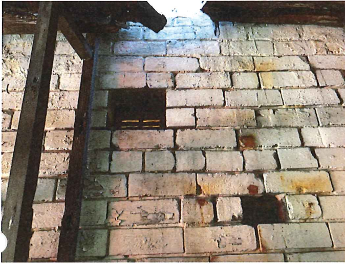
Photo 5 - Internal wall. The walls are typically in poor condition and display significant dilapidation of the lime mortar joints
