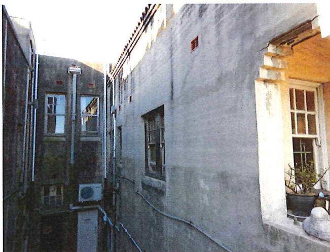
Photo 33 - Facade to internal courtyard. There is evidence of previous repairs to the walls
