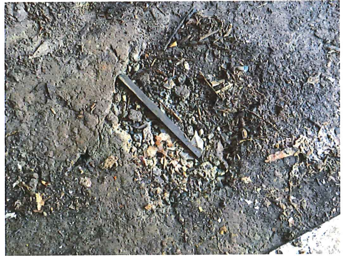
Photo 18 - Damage to ground floor slab
