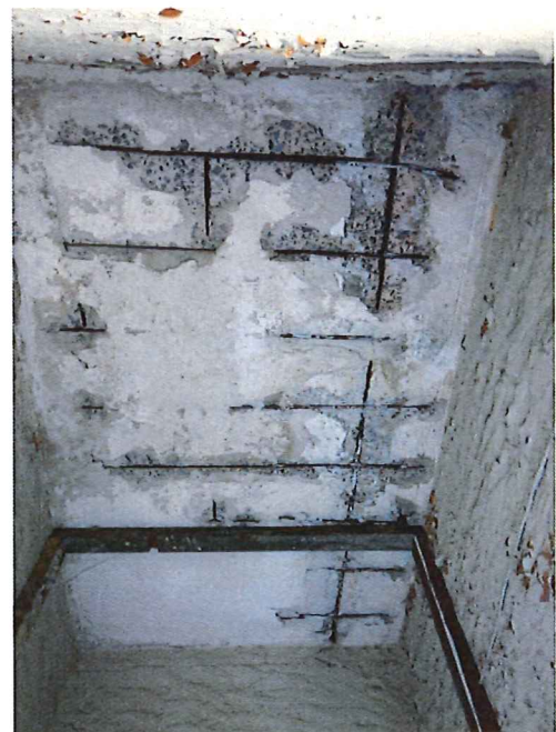
Photo 12 - Evidence of concrete cancer to suspended slabs. This is a significant issue throughout the building through all concrete slabs.
