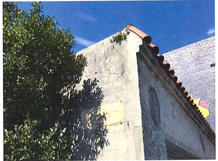
Photo 14 - Cracking to external corner of masonry wall
