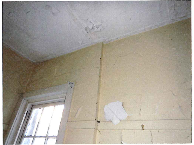
Photo 30 - Evidence of cracking to the internal walls of the upper level apartments
