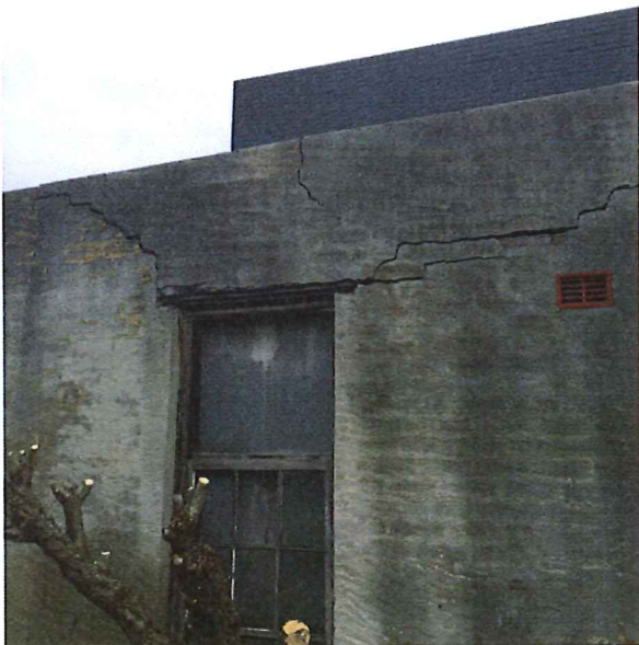
Photo 11 - Damage over window as a result of corroded lintel
