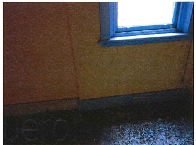
Photo 28 - Evidence of cracking to the internal walls of the upper level apartments
