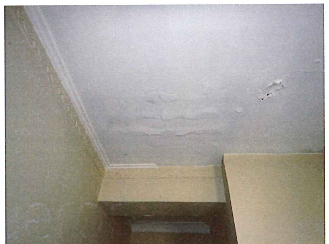
Photo 16 - The undulations in the render to the underside of the slabs are impacted by concrete cancer and spalling of the concrete is immanent
