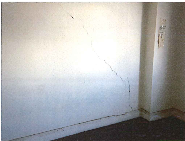
Photo 27 - Evidence of cracking to the internal walls of the upper level apartments
