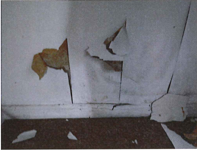
Photo 5 - Example of water damage to walls to lower level apartments. This wall is the rear wall of the bedroom to apartment 2.
