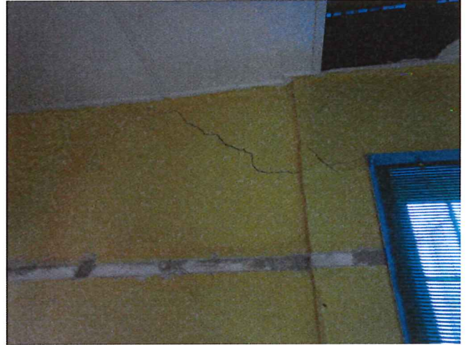
Photo 26 - Evidence of cracking to the internal walls of the upper level apartments
