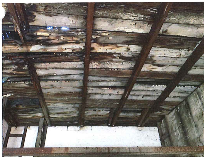
Photo 19 - Significant damage to roof
