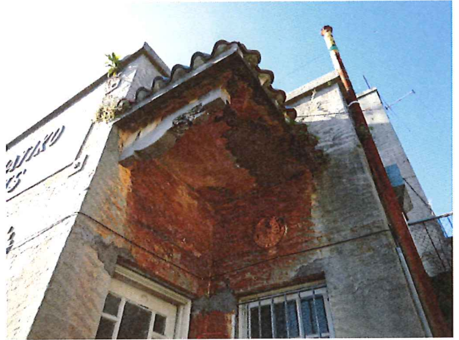
Photo 34 - Concrete cancer to exposed slab details. This is a consistent issue throughout the building
