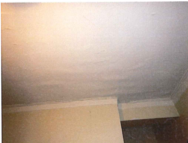
Photo 15 - The undulations in the render to the underside of the slabs are impacted by concrete cancer and spalling of the concrete is immanent
