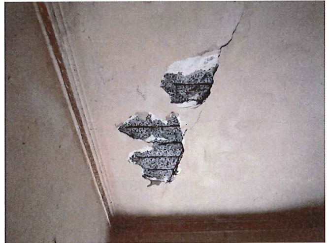
Photo 10 - Evidence of concrete cancer to suspended slabs. This is a significant issue throughout the building through all concrete slabs.
