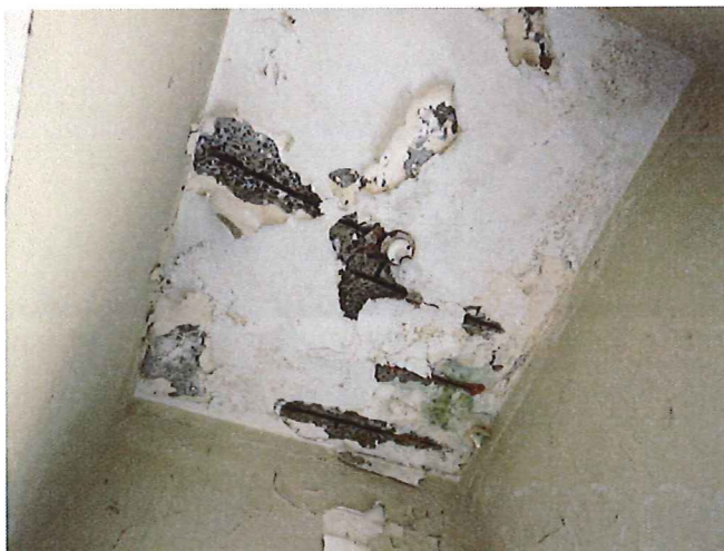
Photo 11 - Evidence of concrete cancer to suspended slabs. This is a significant issue throughout the building through all concrete slabs.
