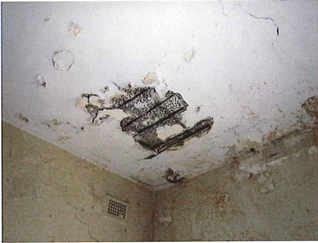
Photo 13 - Evidence of concrete cancer to suspended slabs. This is a significant issue throughout the building through all concrete slabs.
