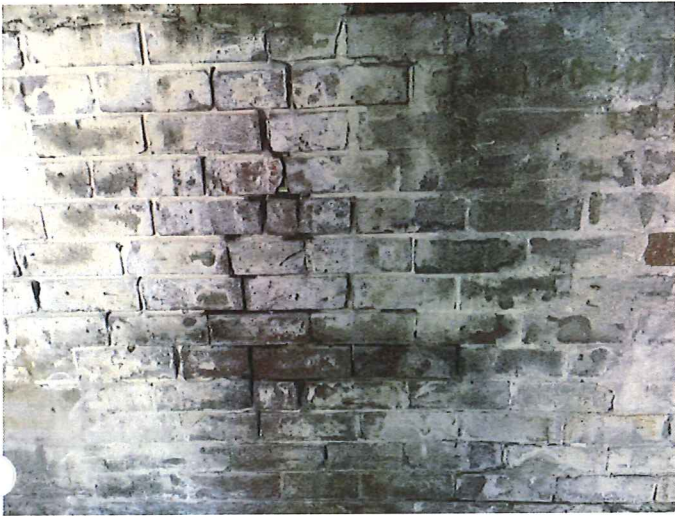
Photo 9 - Deteriorated section of internal wall
