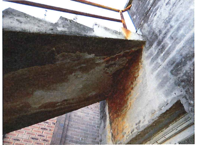
Photo 18 - Evidence of concrete cancer to the underside of the upper level stair leading to the roof top deck
