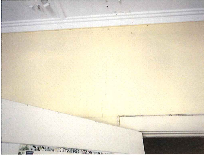
Photo 25 - Evidence of cracking to the internal walls of the upper level apartments
