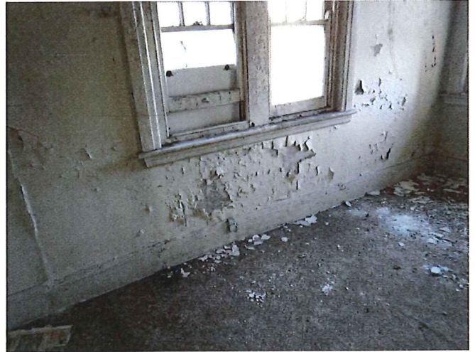
Photo 6 - Example of water damage to walls to lower level apartments. This wall is the side wall of the bedroom to apartment 2.
