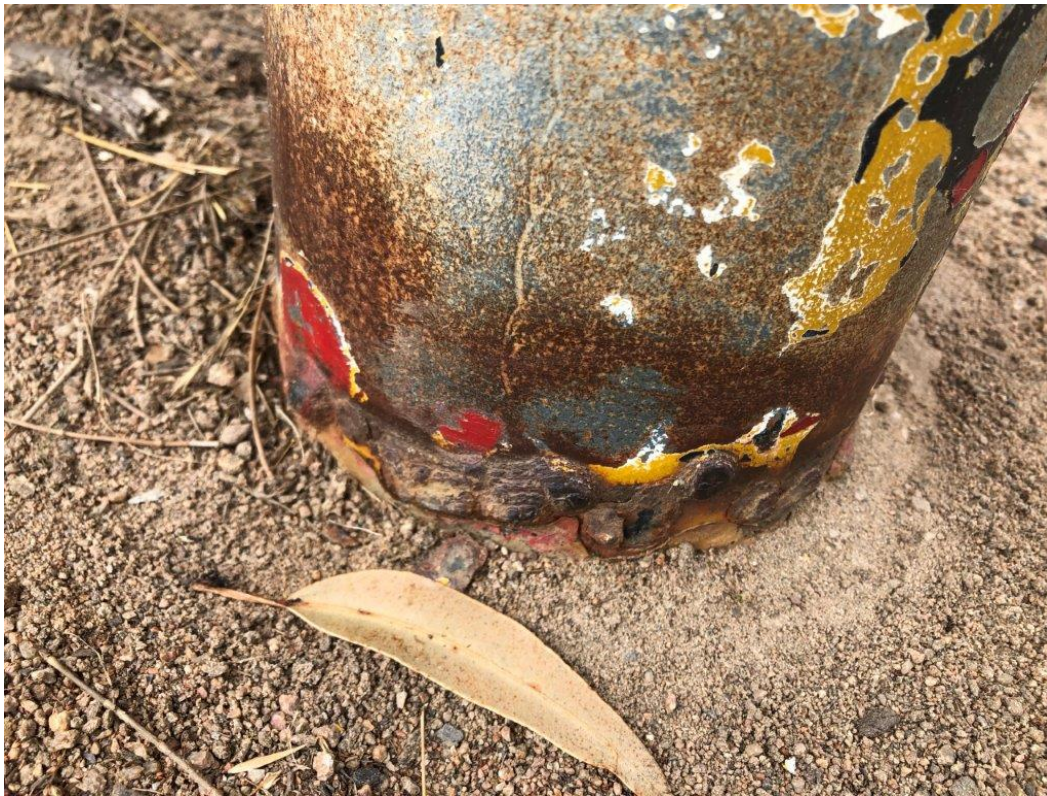
FIG 5. Corrosion (Central Post).
