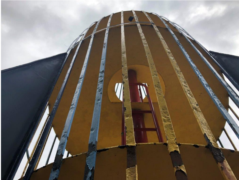
FIG 13. Corrosion (Vertical Bar).
