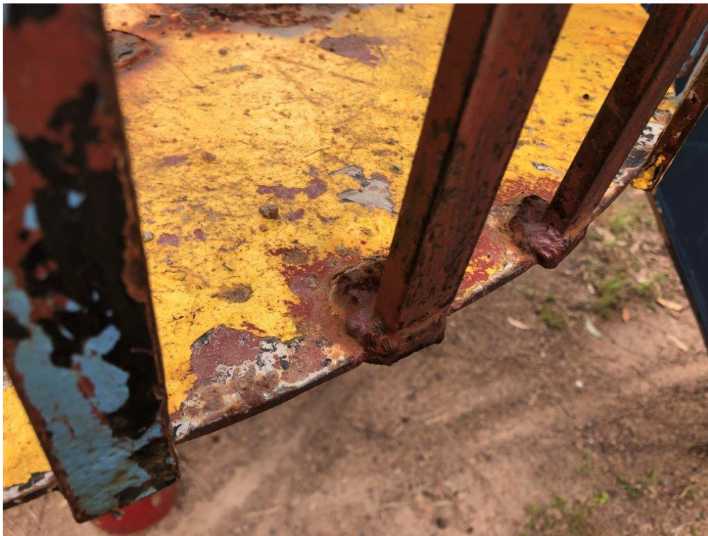
FIG 10. Corrosion (Deck).
