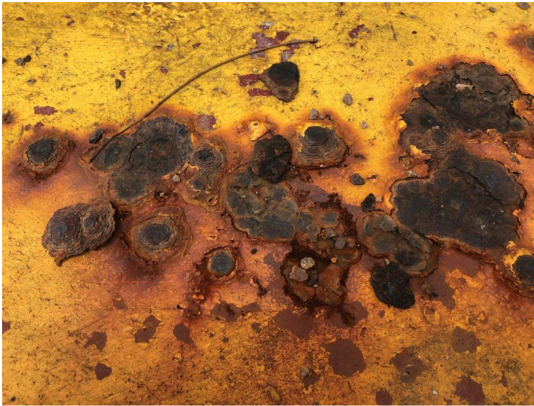
FIG 1. Corrosion (Deck).
