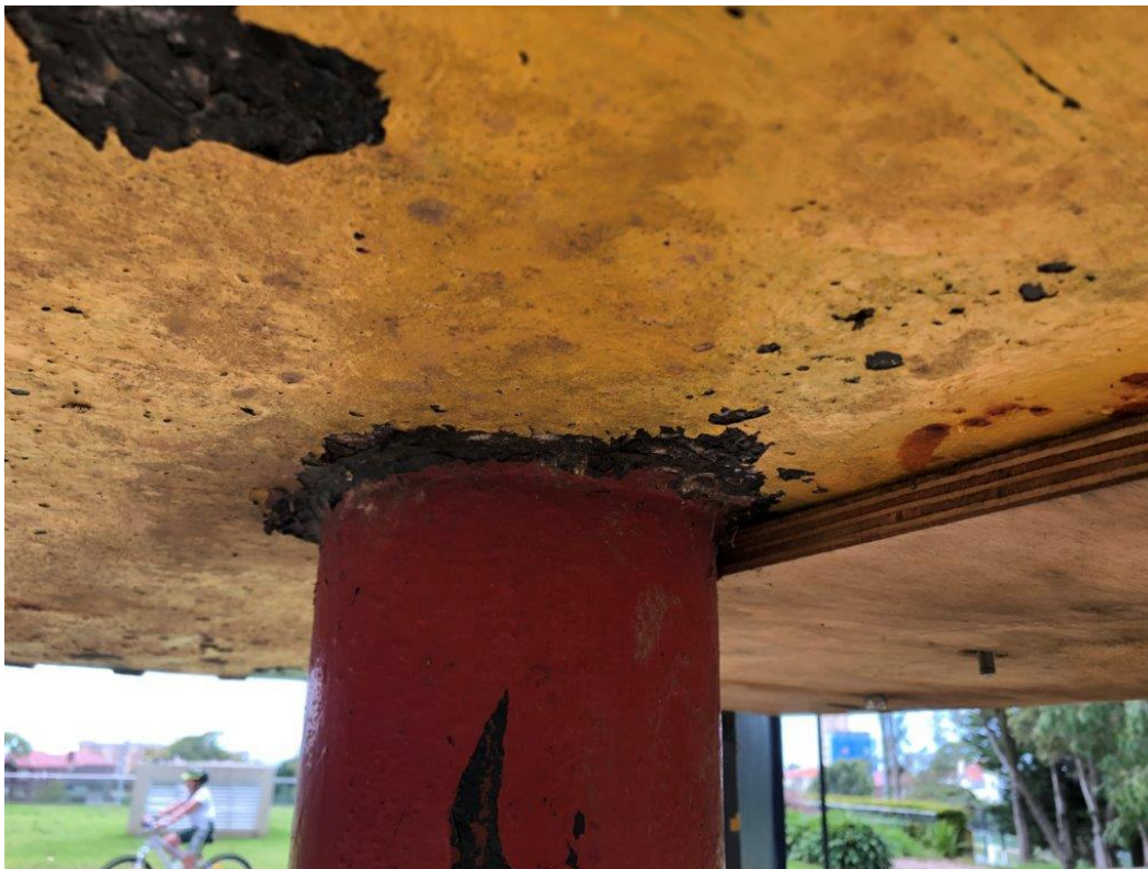
FIG 6. Corrosion (Central Post / Deck Connection).
