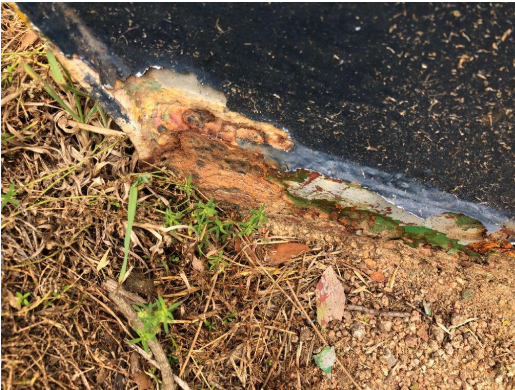
FIG 4. Corrosion (Side Stays at Ground Level).
