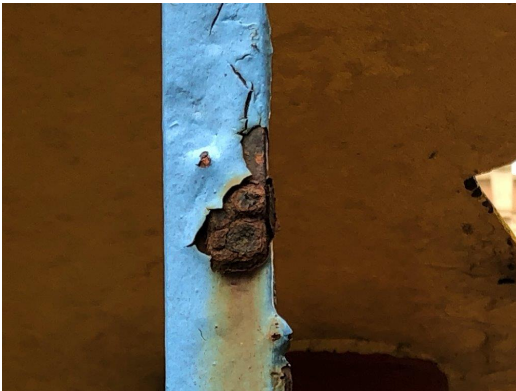
FIG 8. Corrosion (Vertical Bar).
