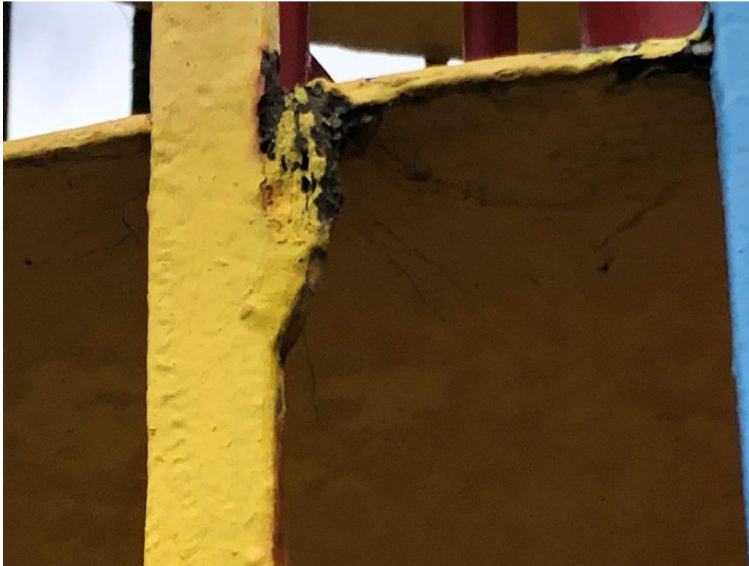
FIG 7. Corrosion (Vertical Bar).
