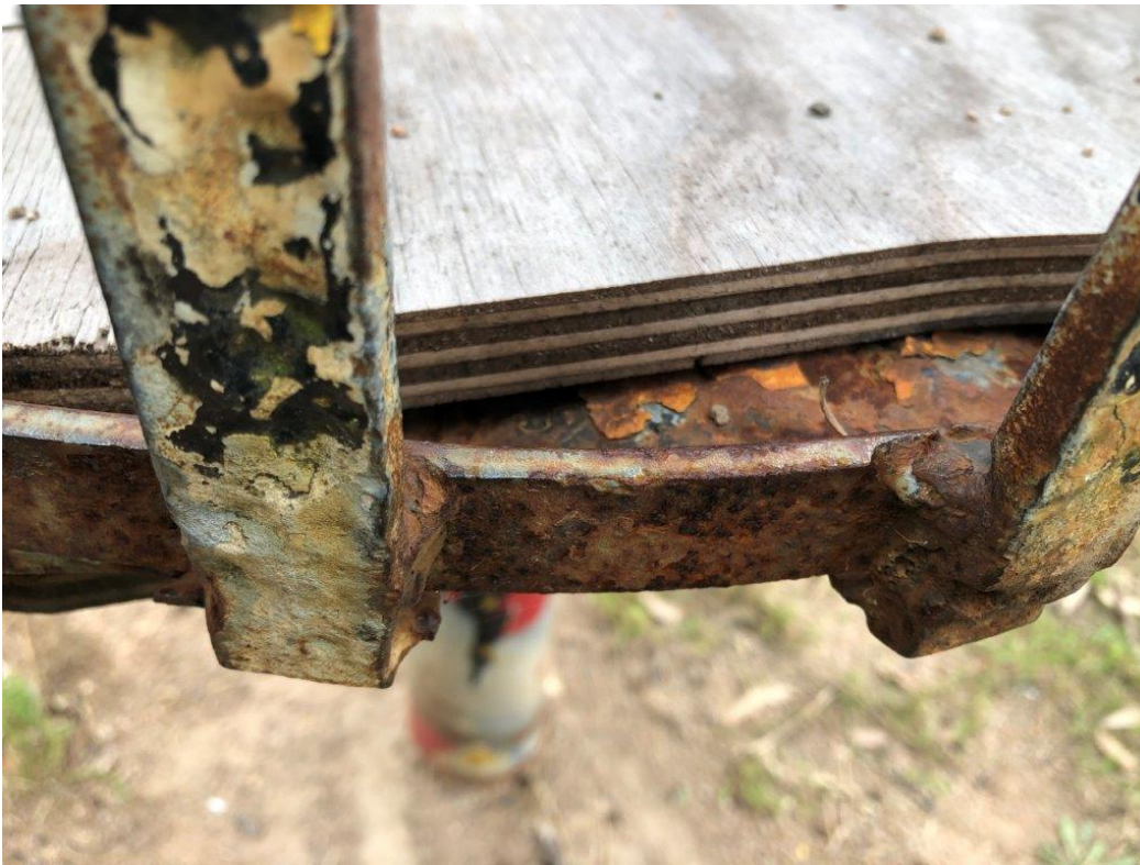
FIG 3. Corrosion (Deck / Bar Connection).
