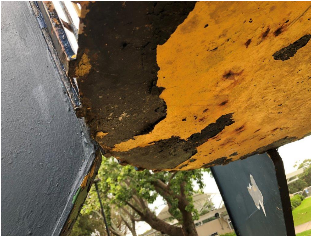
FIG 9. Corrosion (Deck)
