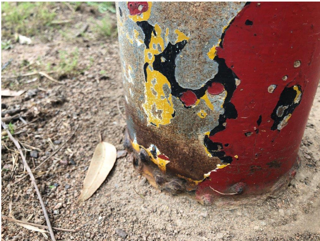
FIG 12. Corrosion (Central Post).
