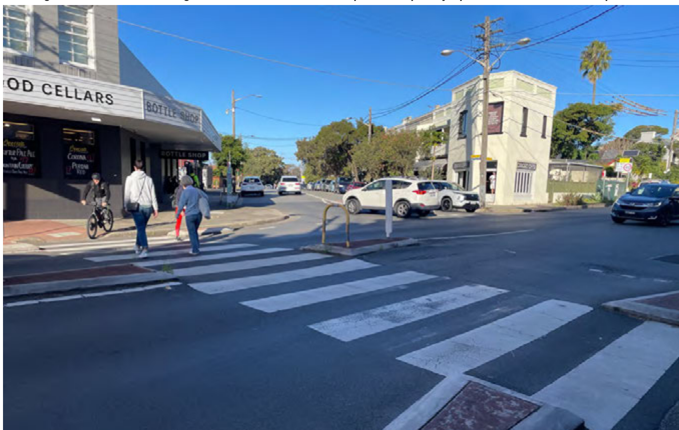
Site image: The existing zebra crossing to the south of the project area is proposed to be upgraded to a raised crossing to enhance ease of use and further calm vehicle traffic
